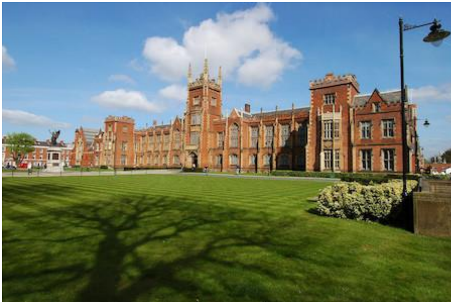
Figure 2. The Lanyon Main Site is open to the public seven days a week.
